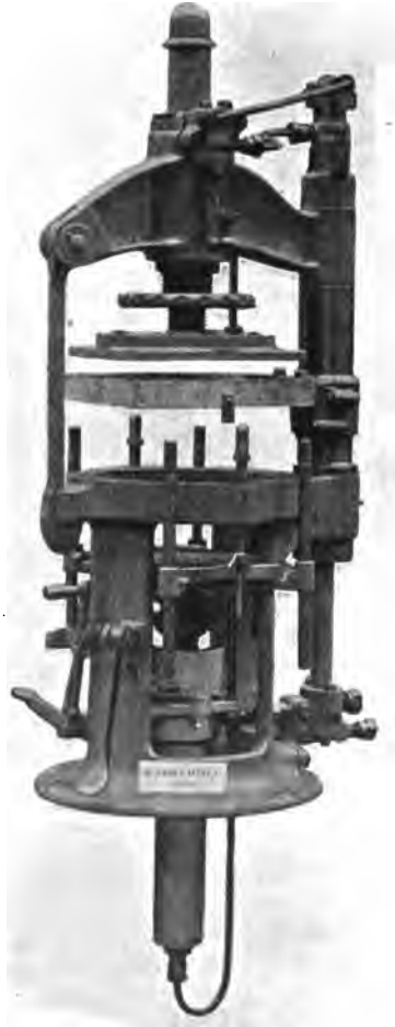
FIG. 276.--Bonvillain Hydraulic Moulding Machine.
